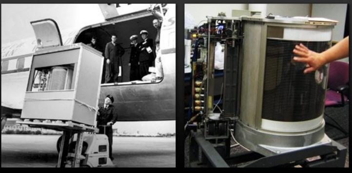
drive—the IBM Model 350 Disk File (came w/IBM 305 RAMAC, 1956).
